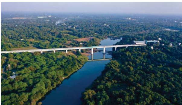
Completion of Bridge on Kharera River, Navsari District, Gujarat
