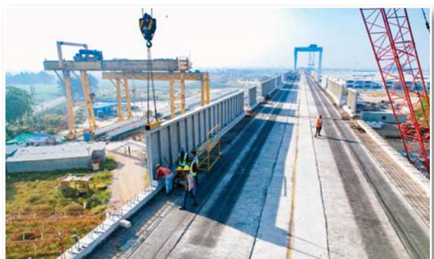
Installation of Noise Barriers in Gujarat
