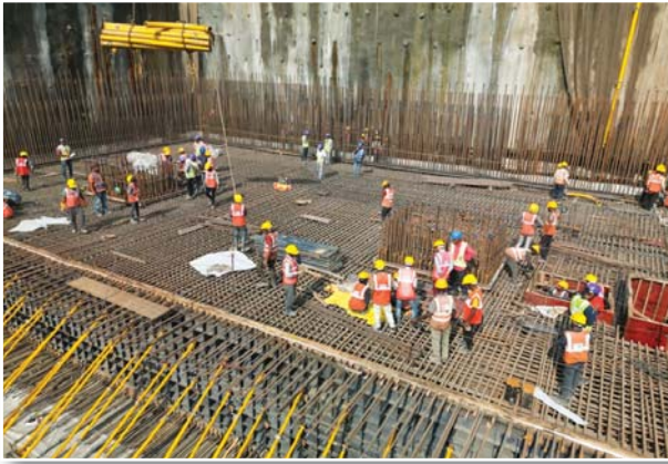
Under-construction Mumbai Bullet Train Station in Maharashtra
