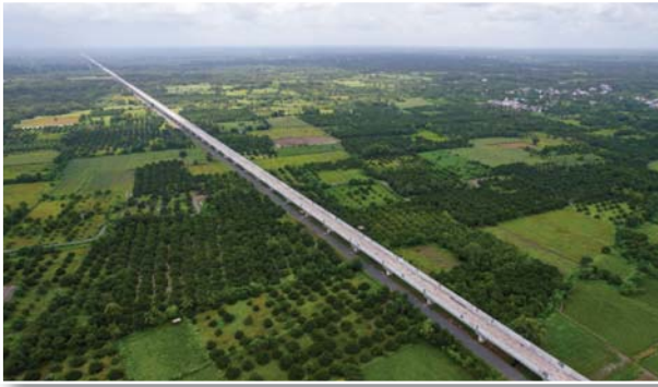
Under-construction Mumbai-Ahmedabad Bullet Train Viaduct
