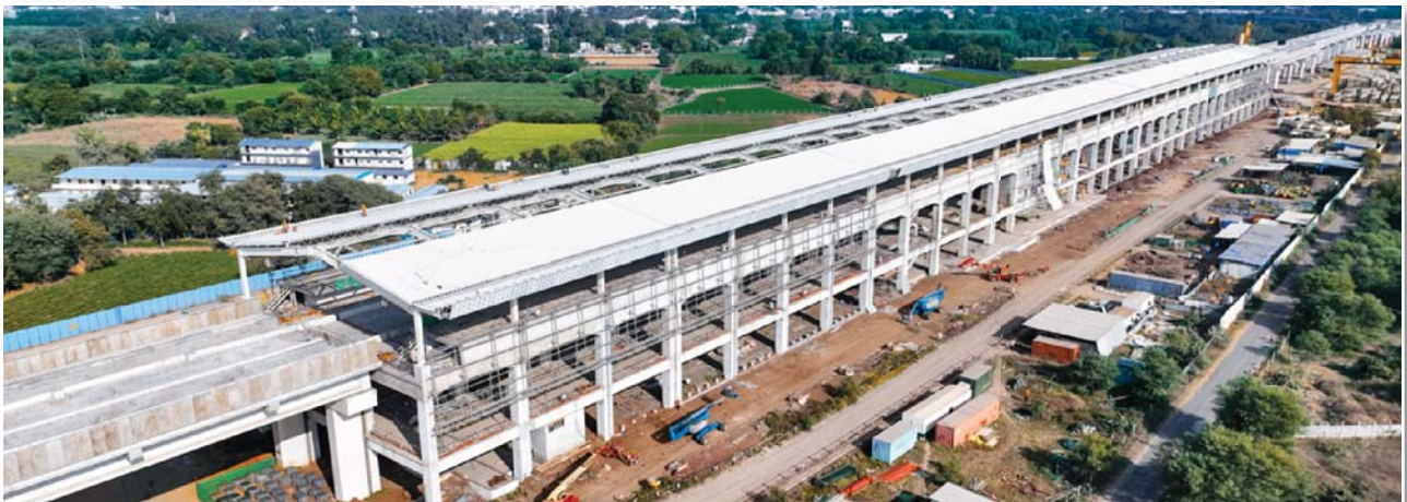
Under-construction Anand Bullet Train Station in Gujarat
